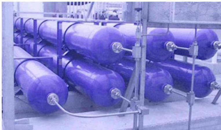
Storage vessels for Hydrogen, Design pressure: 450barg
